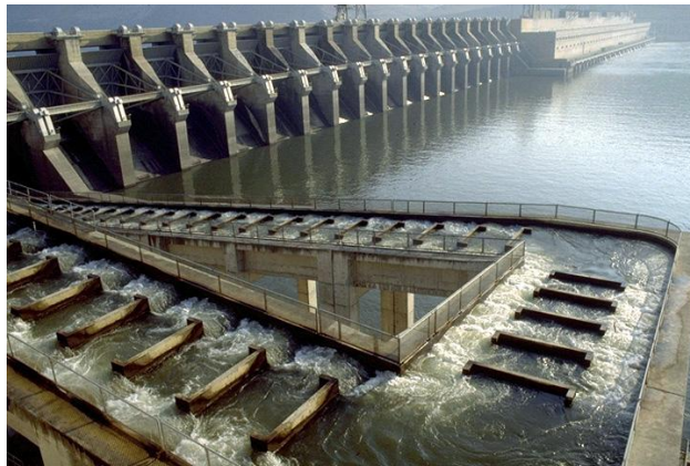
Figure 8: Fish Ladder (Corps of Engineers).
