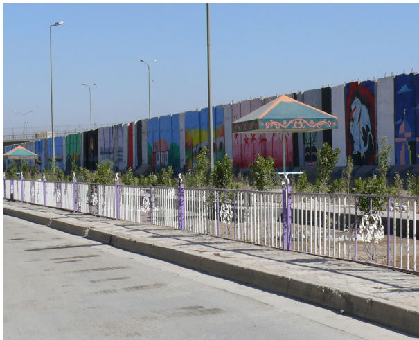
Walls like this one helped to isolate the neighborhoods and made it much more difficult for insurgents to move freely. (Photo by Major Paul Callahan / 1-4 Cavalry)
