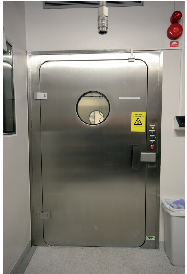
Emergency access door to a BSL4 laboratory
