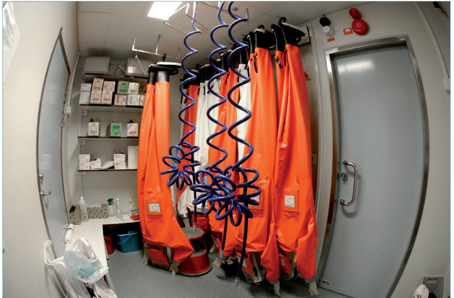
Negative pressure room for suiting up before entering the BSL4 laboratory
