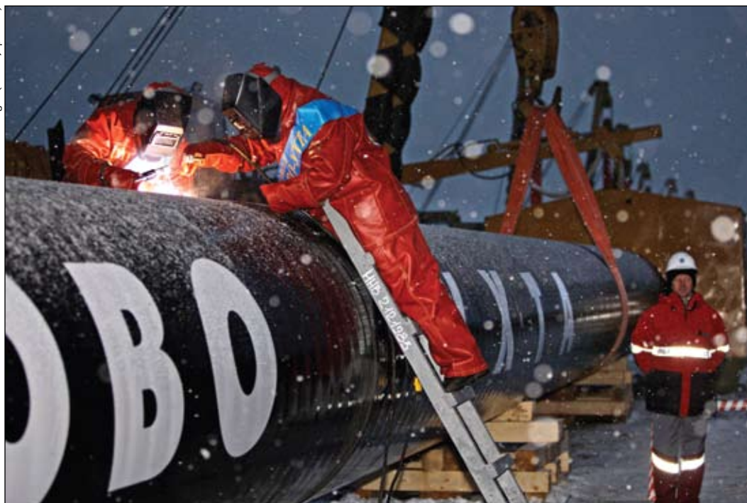
Russian workers weld connection for new pipeline operated by state-run natural gas company Gazprom
