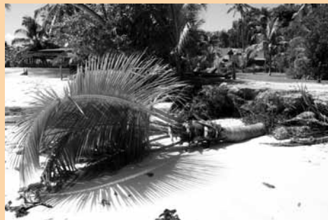
a: Erosion 2001 (before installation)
