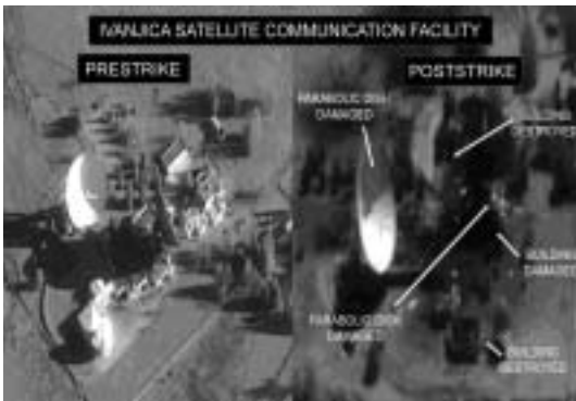
This picture, courtesy of NATO, documents the damage to the satellite antenna and the surrounding infrastructure at Ivanjica satellite ground station.
