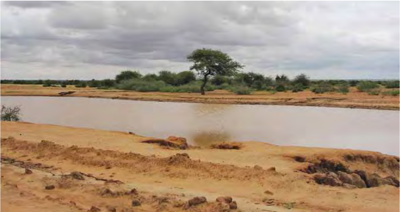
“Hafir” is the Sudanese name for a water reservoir, which is designed to store water runoff after a rainy season.
