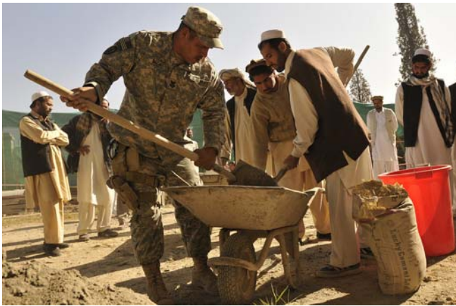
Image 15: U.S. Navy Petty Officer 1st Class Iascc Baca, a builder and Khost Provincial Reconstruction Team engineer, teaches proper mortar mixing techniques to local engineers, construction contractors and foremen during a monthly contractor training session held at the Civil Military Operations Center, Khost, Afghanistan, Nov. 14. Engineers from the Khost PRT provided construction quality assurance training to locals in order to facilitate high quality construction practices in the region. (Photo by U.S. Air Force Staff Sgt. Stephen J. Otero, Khost Provincial Reconstruction Team Public Affairs)
