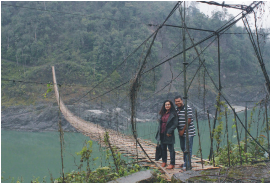
Bridges to border villages, Arunachal Pradesh, March 2011
