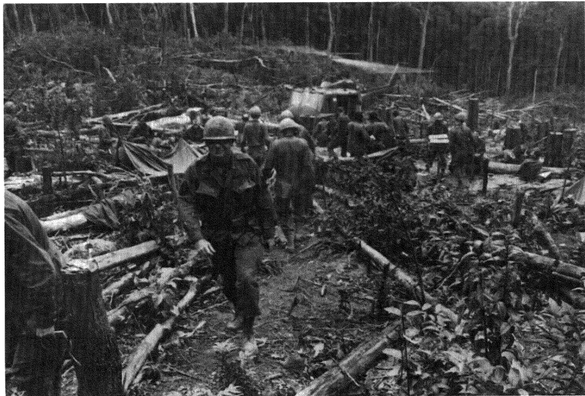
Hastily constructed helipads surrounded by triple canopy rain forests look like holes blasted in green blankets when viewed from above. Observers at ground level see a tangle of felled trees until chain saws complete the clearance process (U.S. Army photographs).
