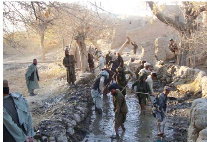
Canal cleaning in Char Chineh District, Uruzgan Province. The survey findings favor irrigation projects tied to long-term agricultural benefits.
