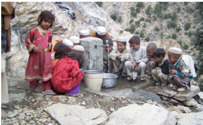
An LGCD water pipe scheme in Khogyani, Nangarhar Province.
