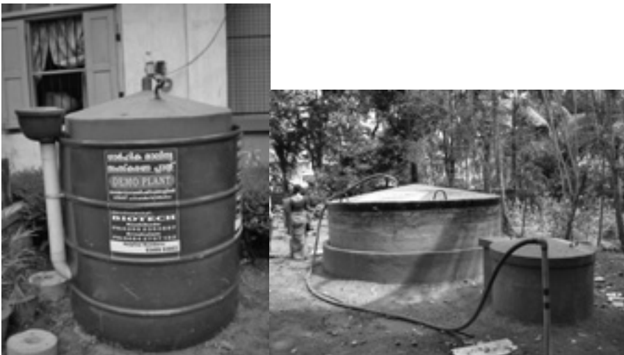
Figure 3.15 Floating drum digester tanks used in India
