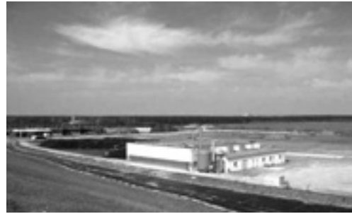
Figure IV.3 A BEKON dry digestion plant
