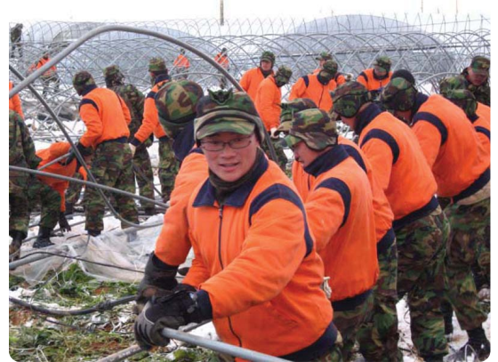
▲ Restoration of a greenhouse after the snowstorm
