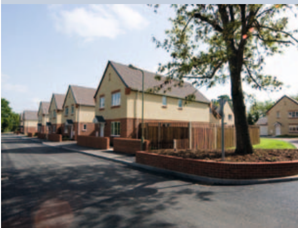
Modernised Service Family Accommodation
