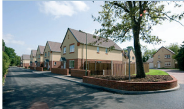
A street of modernised Service Family Accommodation (SFA)
