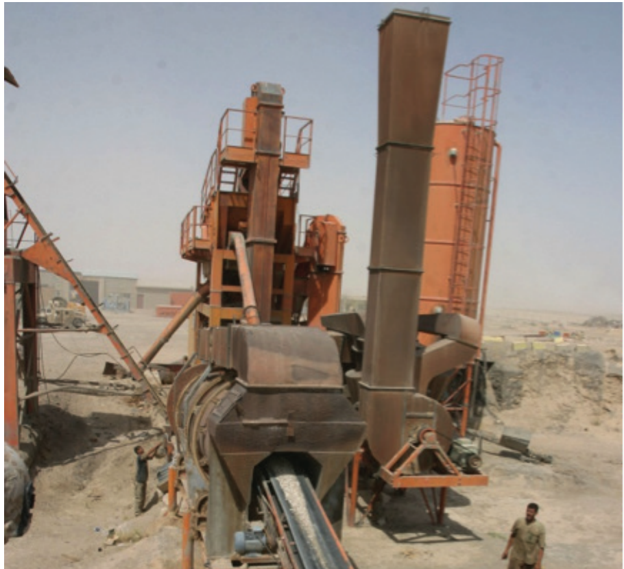
FIGURE 3: AN ASPHALT FACTORY IN RAMADI, IRAQ.
