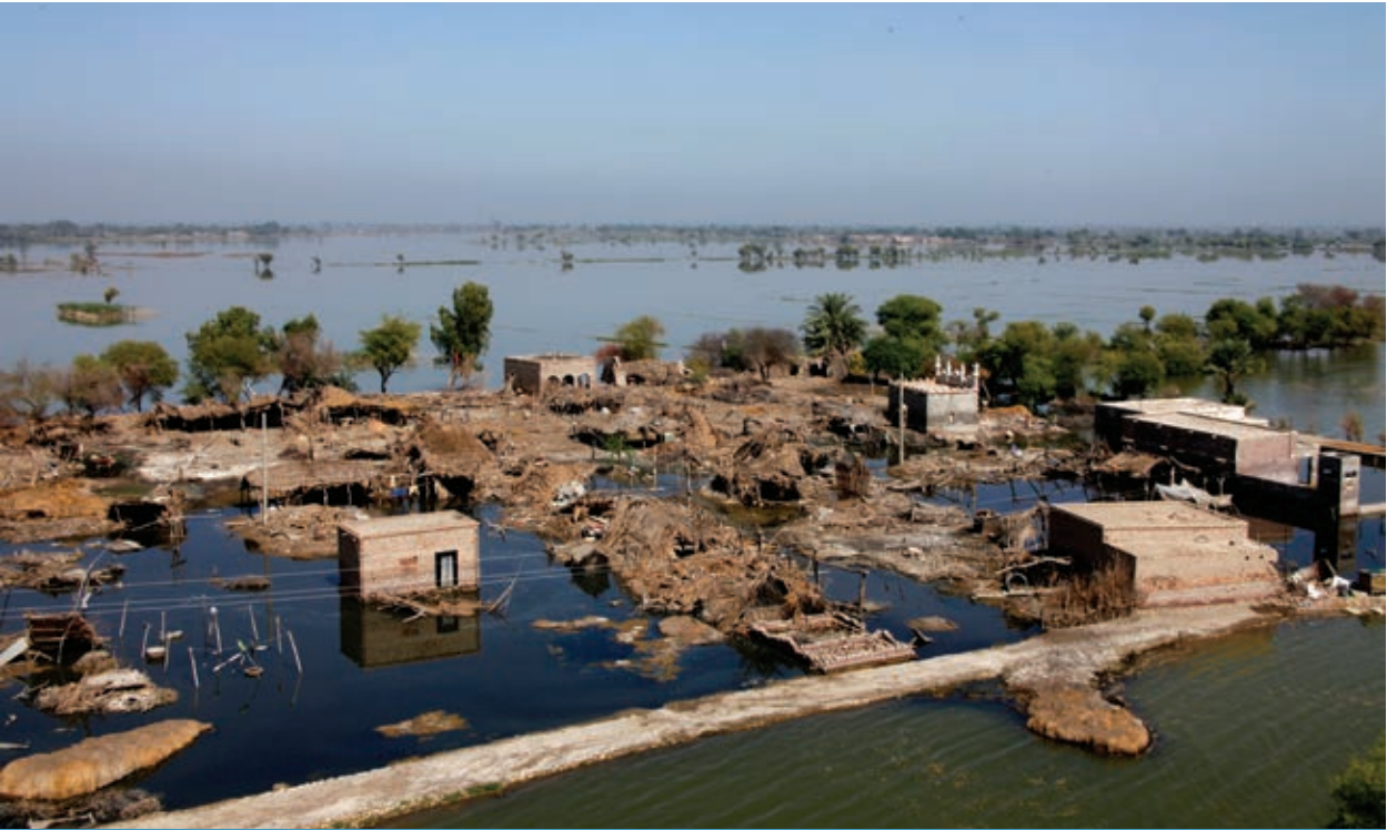
Flood damage in Sindh Province, Pakistan, October 2010.
