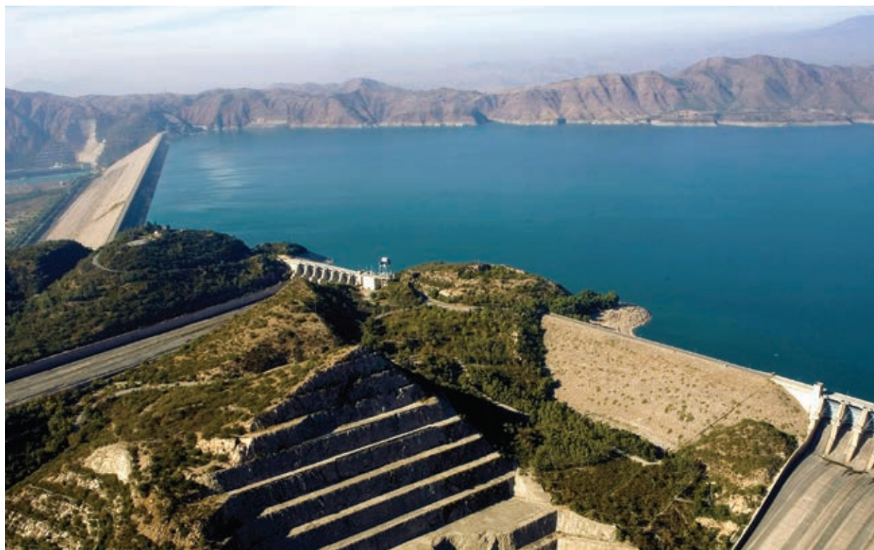
Tarbela Dam, Haripur District, Hazara Division, Khyber Pakhtunkhwa, Pakistan.
