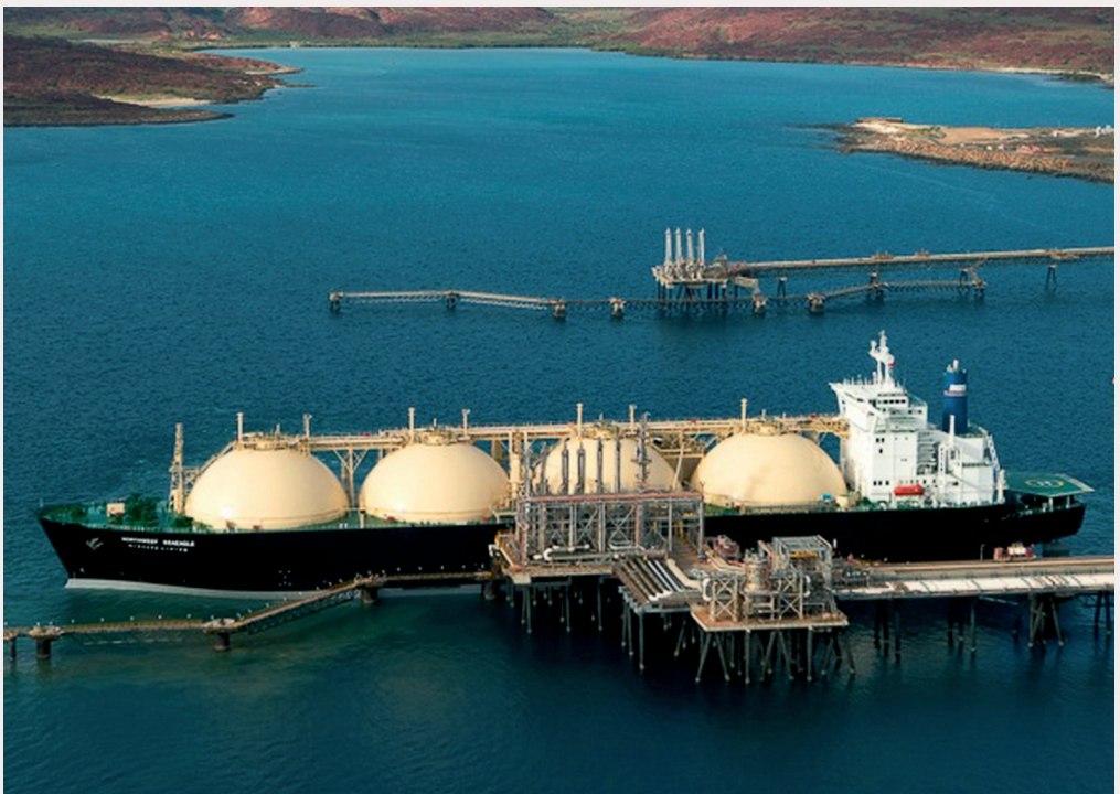
LNG (liquefied natural gas) tanker at the Karratha gas plant loading terminal, Western Australia © Woodside Energy Ltd.
