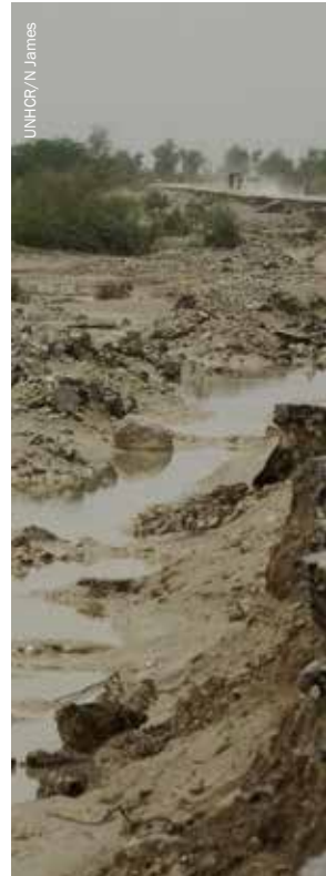
Road damaged by floods in Balochistan, Pakistan, 2010.
