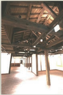
Roof trusses of Shirakabe Heisya Public Historical Center (GSDf Camp Shibata)
