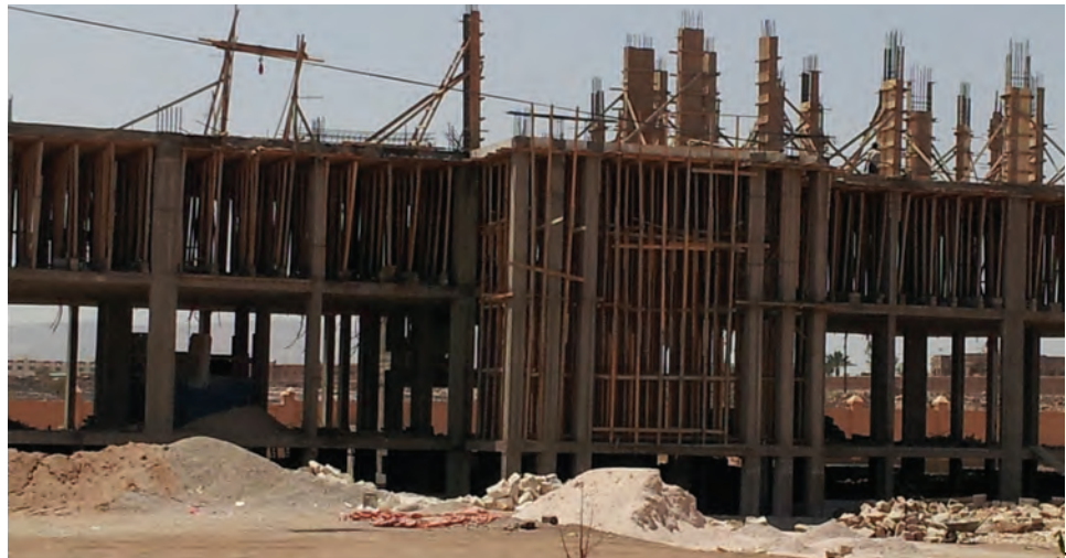
Photo 4. New judicial complex under construction in Taiz.
