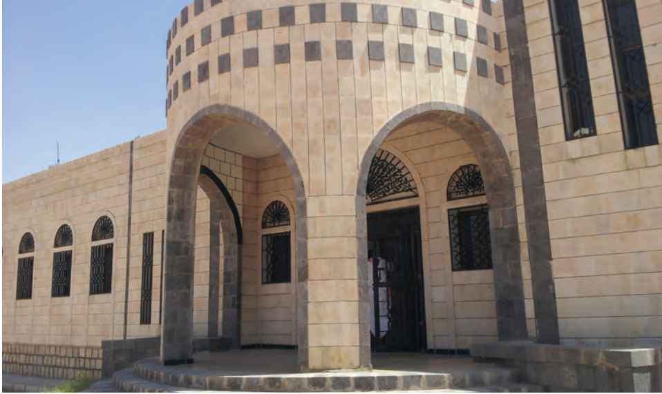
Photo A6.7 Marib court of appeals and Marib City's primary court.
