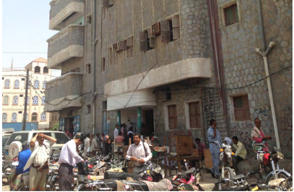
Photo A6.4 Hodeida North and circuit courts.
