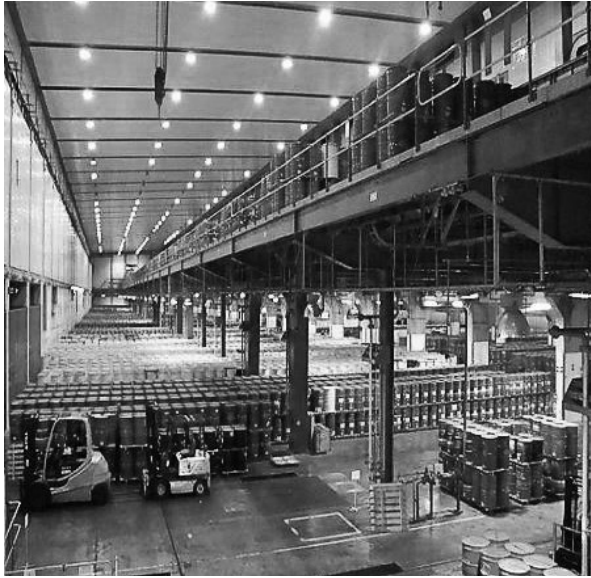
Figure 9-1. Temporary Storage of Waste Drums in a Decommissioned Enrichment Plant. 7
