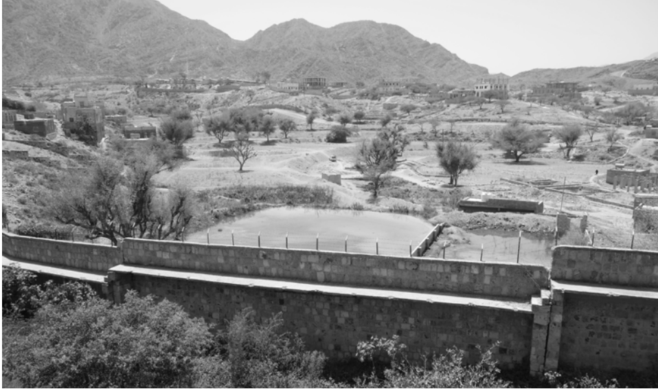
Photo 6. Sewage Leak Along Perimeter Wall, Taiz Central
