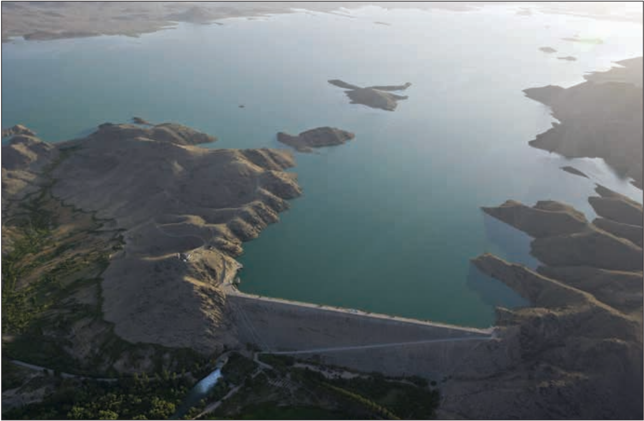
The Dahla Dam
