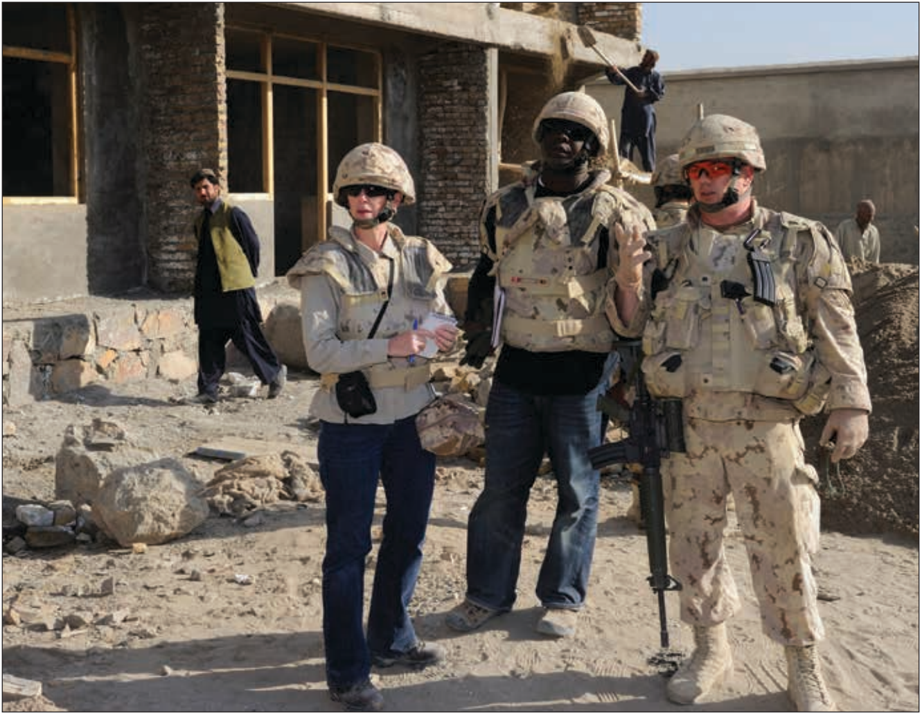
Barbara Humick and Mark Duah from CIDA with a CF member assessing construction progress in Kandahar, 26 November 2010.
