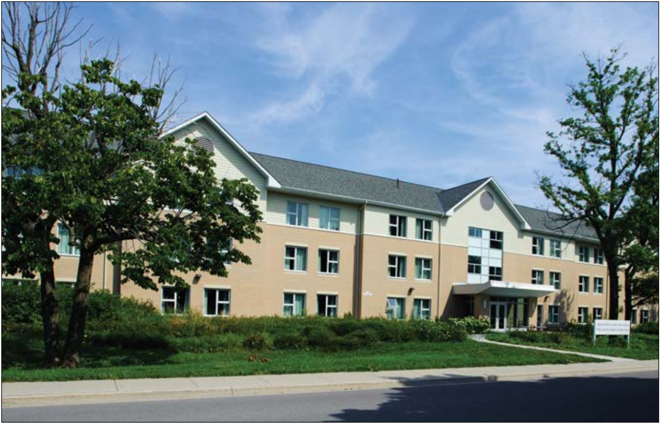
The Vimy Training Quarters in Kingston is a three-storey, 5160 square metre military residential building, modeled as a modest hotel, and it is an example of a DND Green Globes Building.
