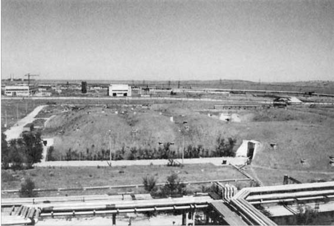
Buildings 251-252, used to store finished products
