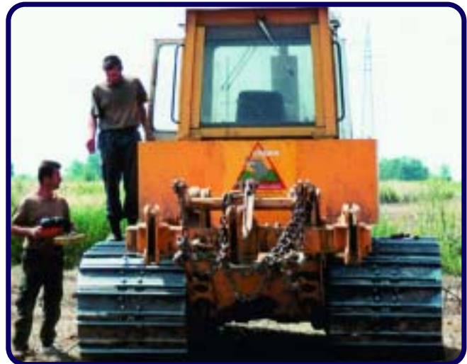
Figure 3 The third machine with the attached rake
