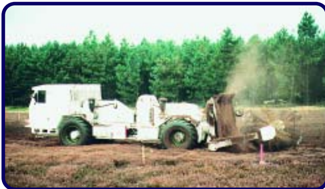
Figure 4 The Hydrema 910 MCV in operation
