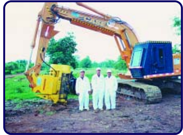
Figure 3 PRO MAC BDM 48 maintenance team
