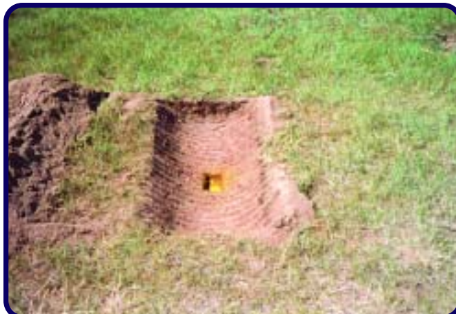
Figure 4 Example of a bite from the PRO MAC BDM 48
