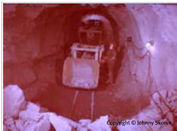
Fig. 7. Excavation in tunnel
