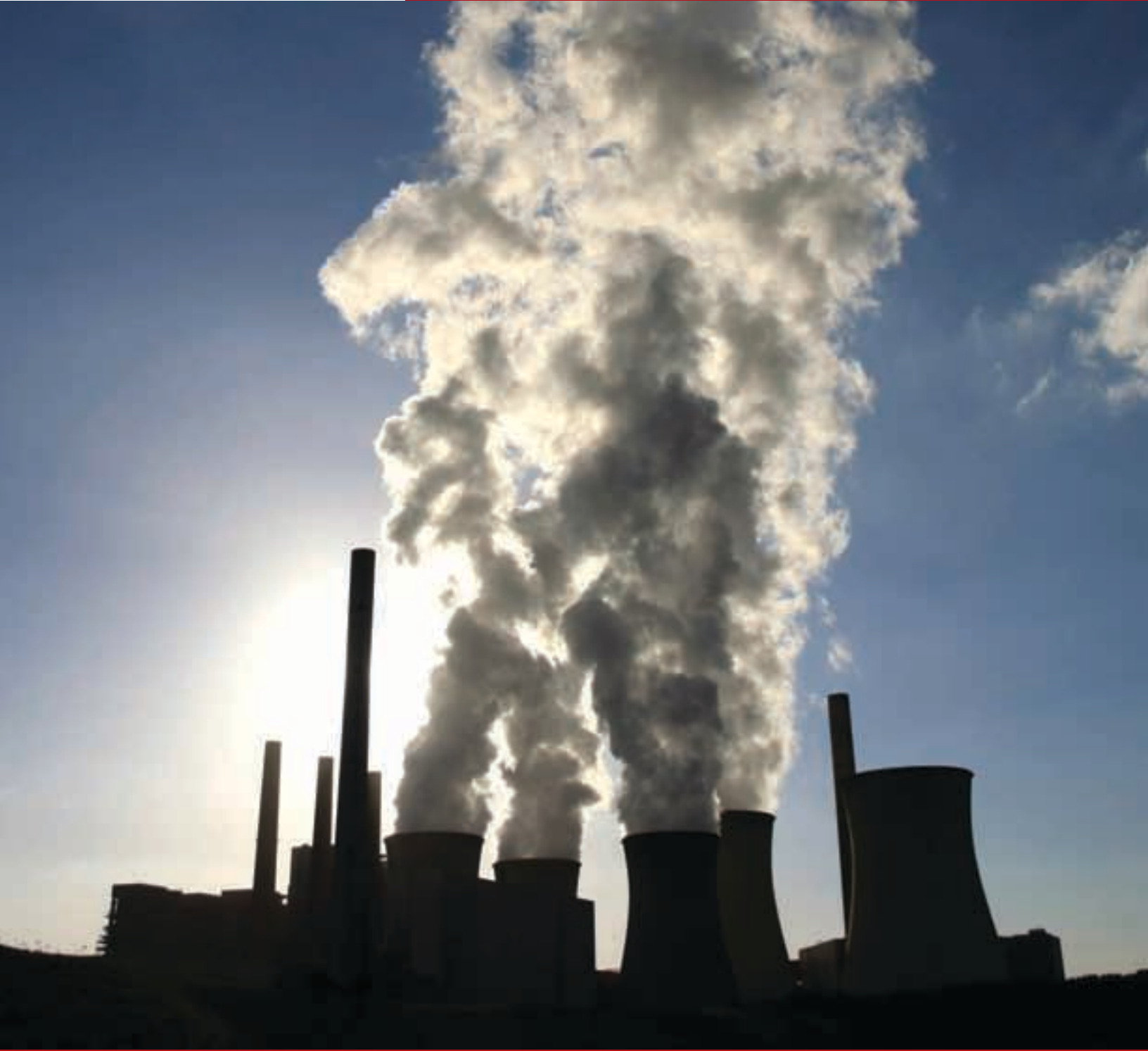
LOCATION: West Germany — Silhouette of the Neurath Power Plant.
