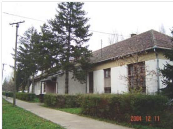
Site 1 – Building I
