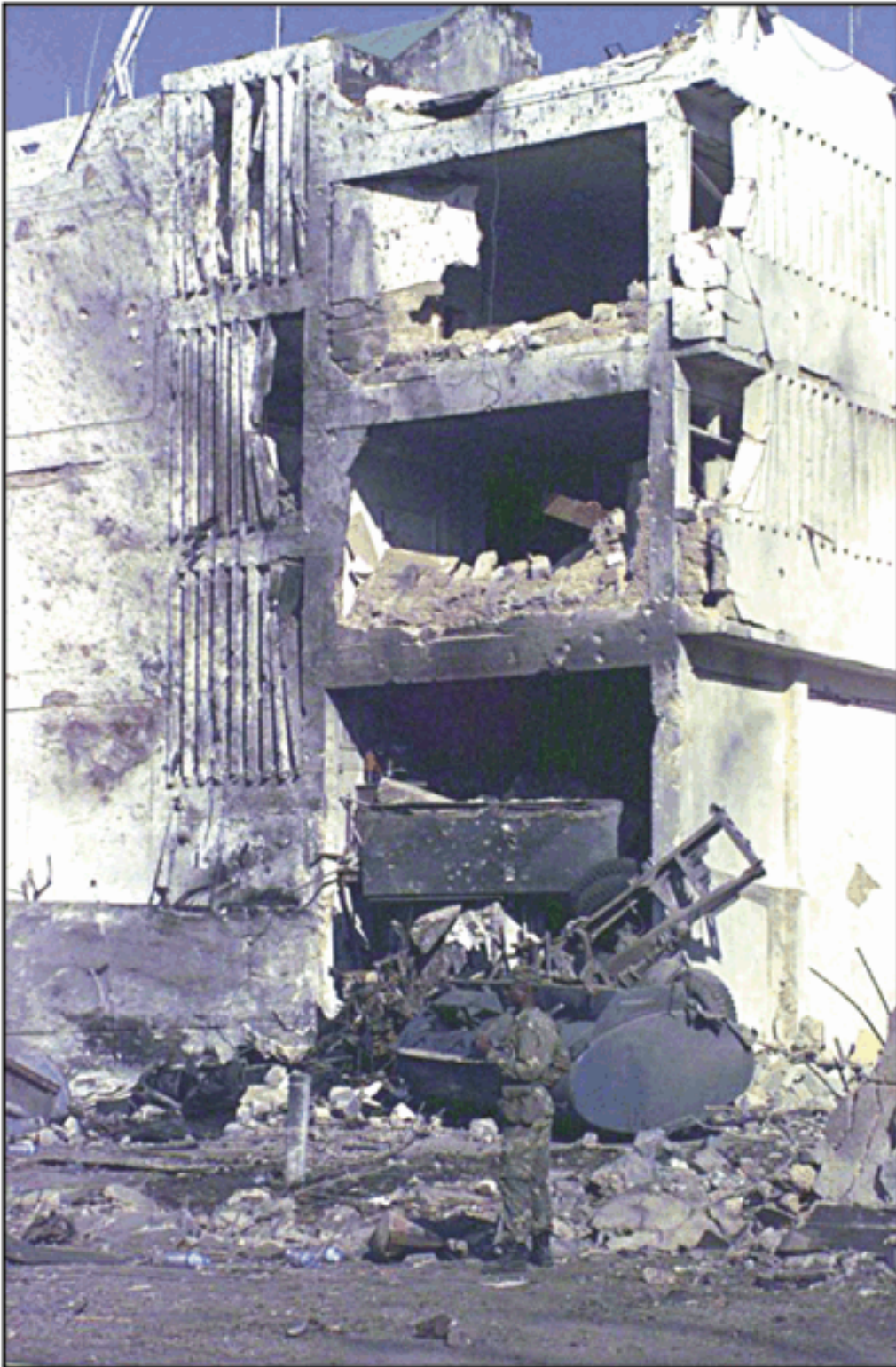
Exterior of US Embassy building in Dar es Salaam after bombing, 7 August.
