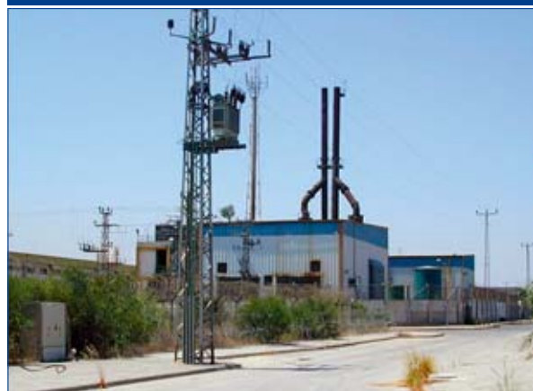
Figure 2.10: IPP Power Station in the EIE
