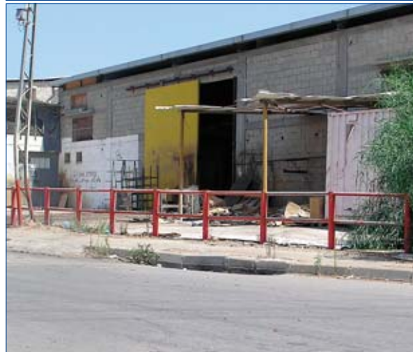
Figure 2.5: Lack of Zoning, Service Entries, or Logistics Infrastructure
