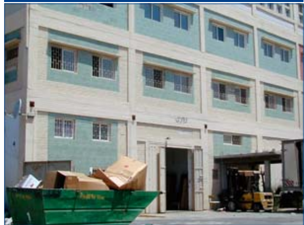
Figure 2.3: In-situ Concrete Structure
