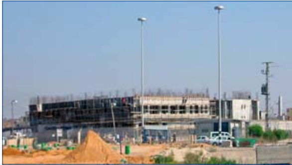
Figure 2.22: New Erez Passenger Terminal under Construction (June 2005)
