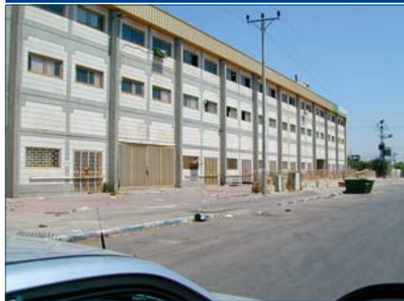
Figure 2.2: Prefabricated Industrial Building
